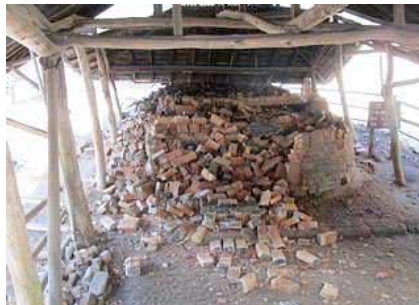
The Hamada kiln after the Mar. 11 earthquake in north eastern Japan.
