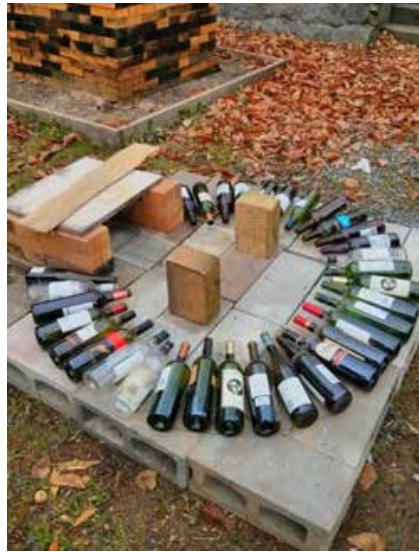
LEFT: Laying out the base and first course.
